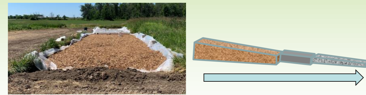
Figure 5. Hybrid Swale: Installed (L); 3 cells: woodchips, slag, gravel (R)
